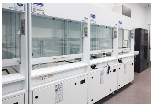
Four high specification fixed fume cupboards
