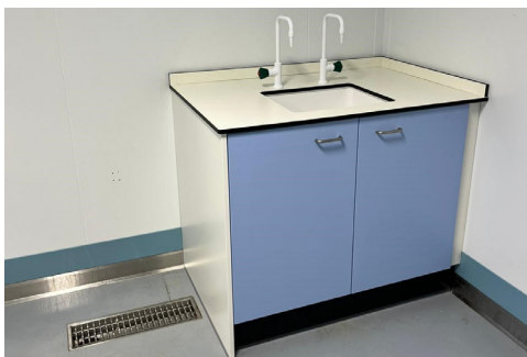
Fitted sink unit designed to fit around floor drain
