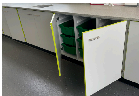
Perimeter benching with contrast door edging
