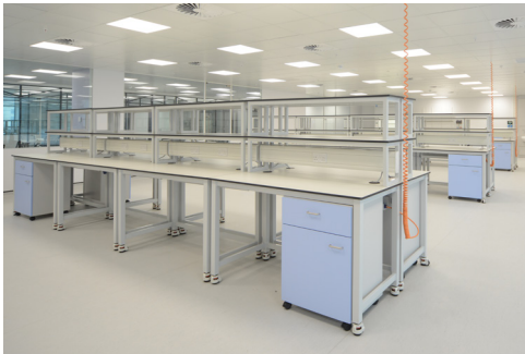
Super large lab - power connections to workstations
