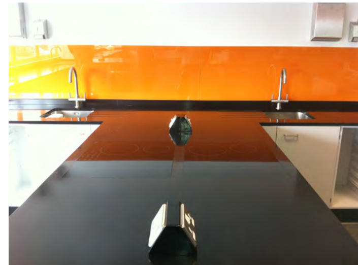
Contrast hygienic cladding - avoid fitting next to a heat source
