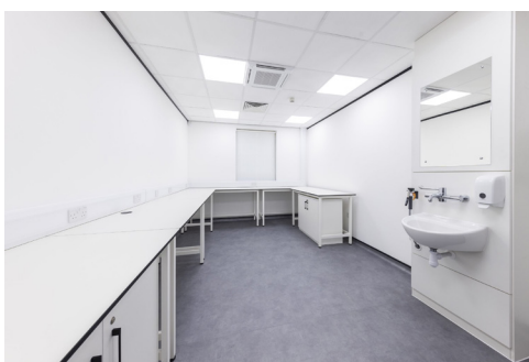
Lab fitted with perimeter benching and IPS unit
