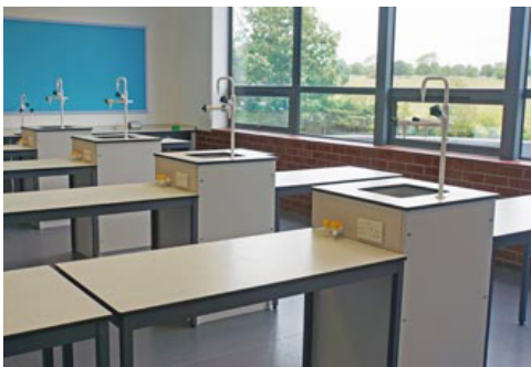
Serviced bollards with loose tables
