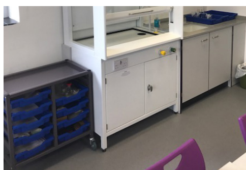
Fixed fume cupboard & mobile tray storage
