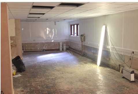
Work in progress showing structural pillars
