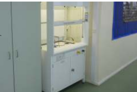
Fixed fume cupboard
