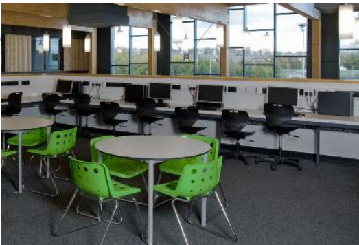
Wall mounted trunking
