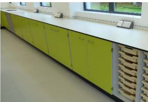
Perimeter Trespa benching with lime doors.
